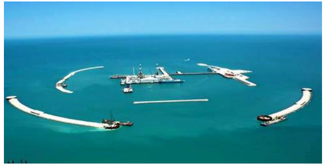
FIG. 1. Multiple arc-shaped breakwaters applied in the Kashagan Oilfield in Caspian Sea, Kazakhstan.
