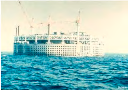
Fig. 1. Ekofisk gravity structure in the North Sea (Song and Tao, 2007).
